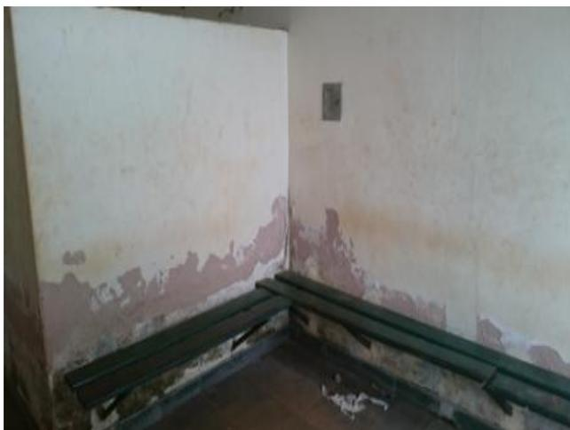
**Foto 11: Pintura descascando**
